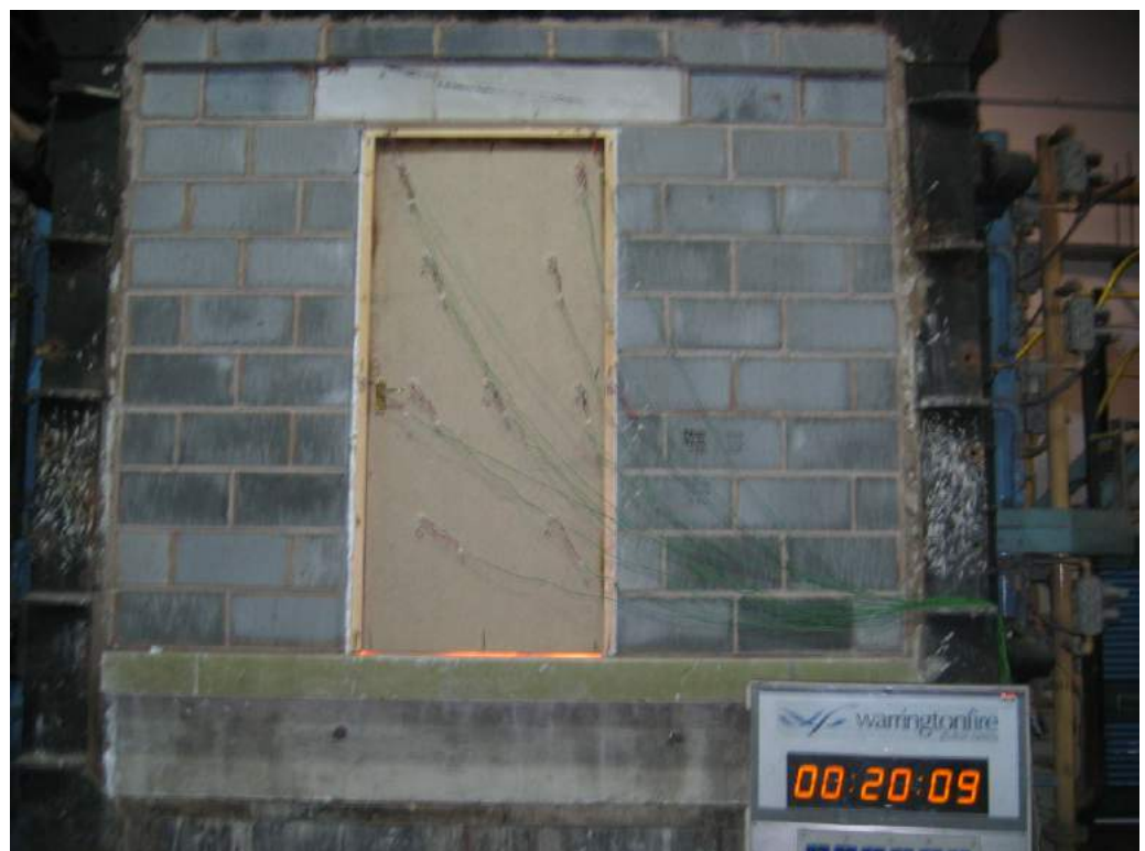
The unexposed face of the doorset after 20 minutes of testing
